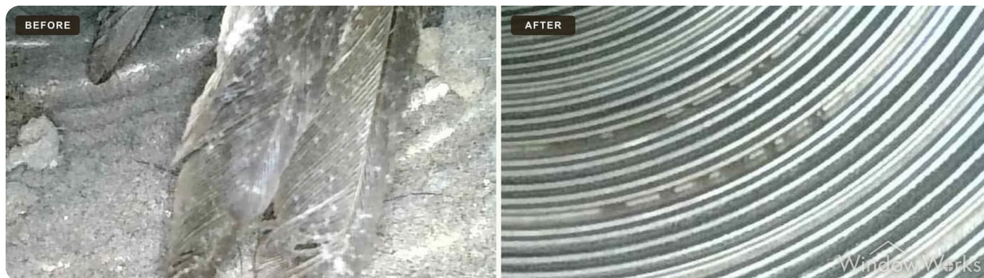
A bird that got in through a failed vent flap and could not get back out. The homeowner's only symptom was slow drying.
