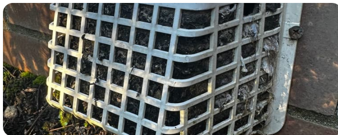
A guard fitted to the exterior hood after clearing the duct.
